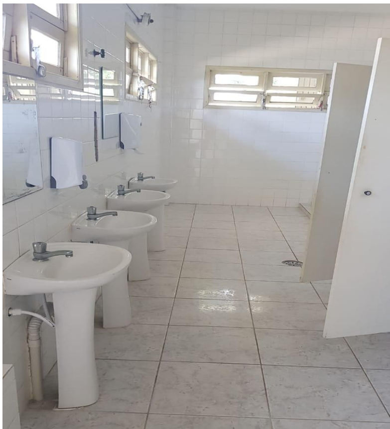
Shower - General View
