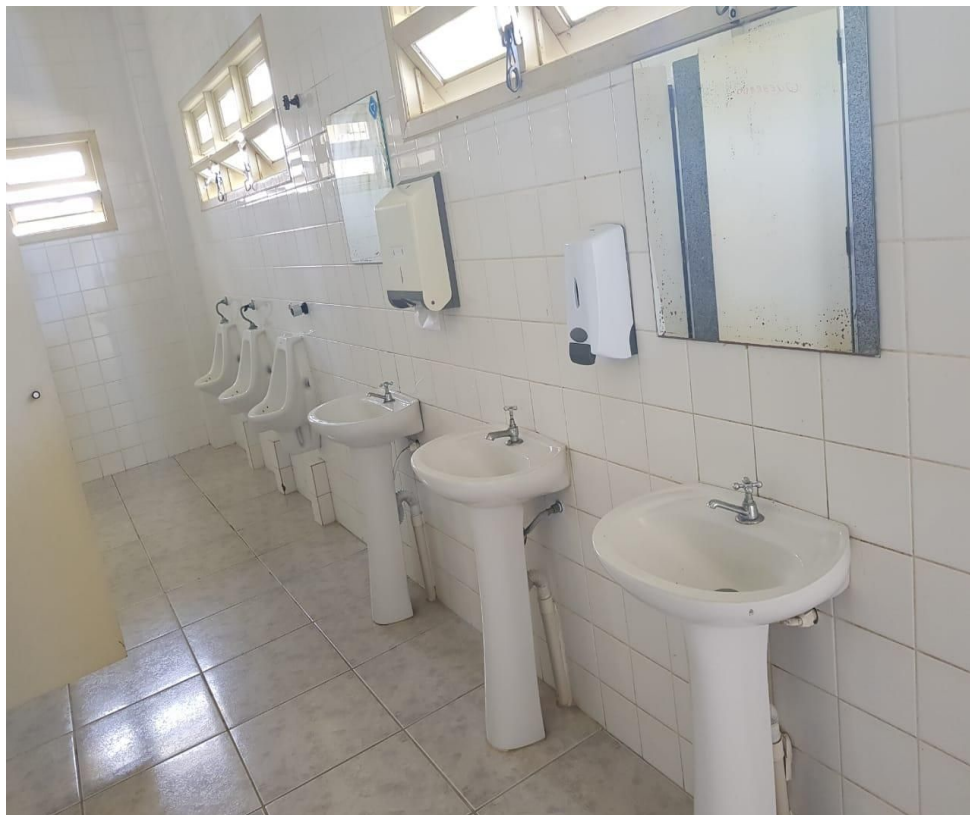
Showers - General View
